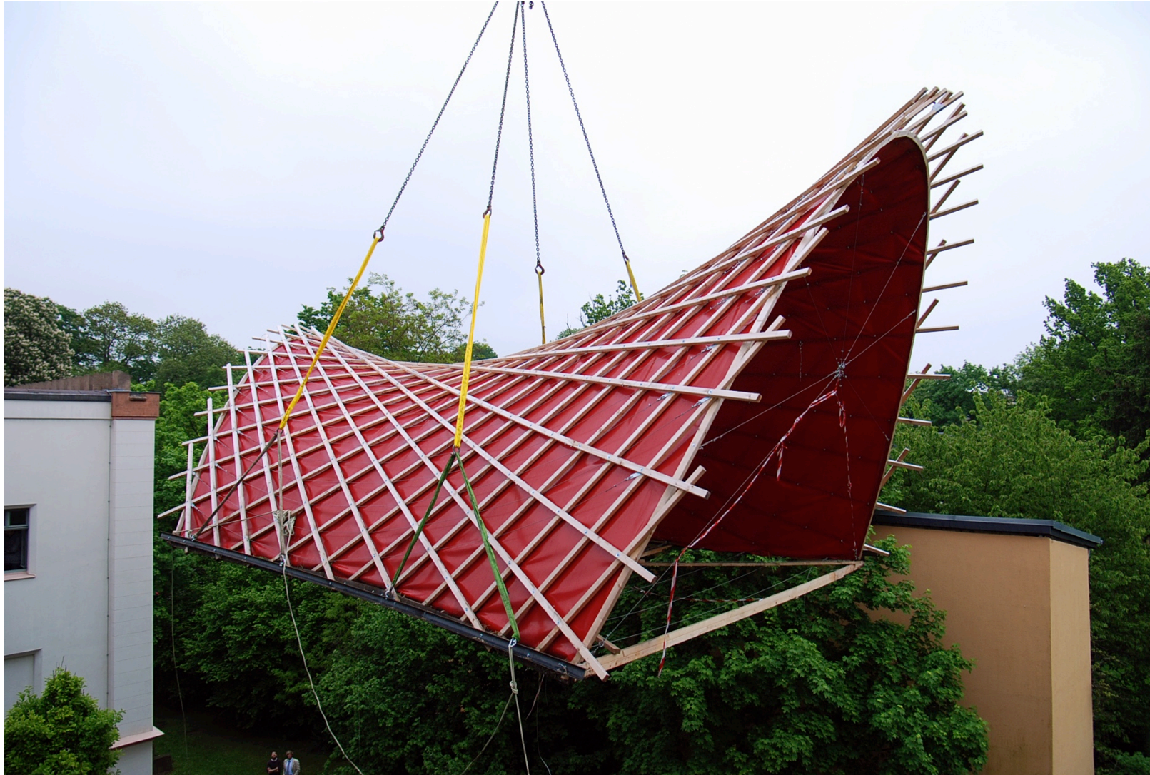
SCREENHAUS SOLAR Germany Land of Ideas award 2010
